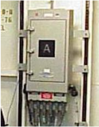
Figure 20: Connectorized Legacy Power Panel
